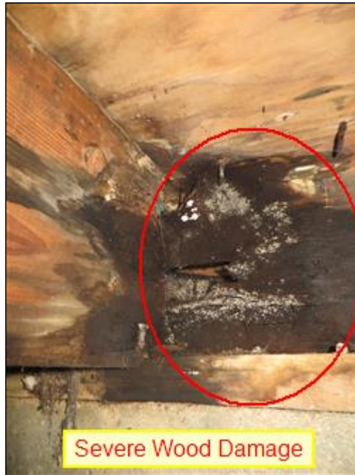
Severe Wood Damage
