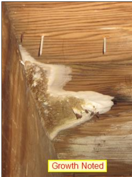
Severe Wood Damage
