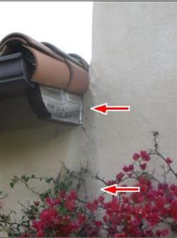
(3) Sprinklers Hit House. There were a few areas of stucco discoloration. It appears the the exterior sprinklers are hitting the house at some locations. It is important to keep all water away from the house and foundation. Sprinklers that hit the house can cause the stucco to fail and delaminate. It is recommended that the sprinklers be adjusted or changed to drip irrigation.
