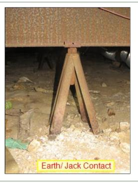
(2) Minor/ Moderate Jack Damage. There are a few jacks at the underside of the home that had some damage. It is recommended that the jacks at the underside of the house be further evaluated for damage and that all damaged jacks be repaired or replaced as needed by a licensed contractor.
