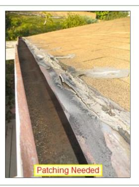
(4) No Overhang at Rake. Roof coverings should extend off the roof by a minimum of 1/4 inch. This was not observed in all area of the overhang. This is to allow the water to drip off the roof and not damage the fascia or eave boards. When roof is replaced, it is recommended that an drip edge be installed around perimeter of house.
