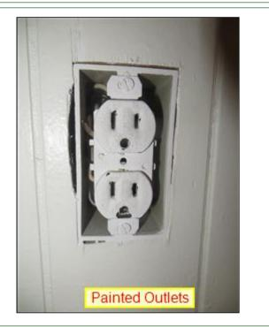
(3) Missing Outlet Covers. There are several missing covers in some of the rooms. Missing faceplates expose electrical parts of receptacle outlets, and switches creating a potential shock hazard. It was noted that these covers were present, but appeared to be off for painting purposes. For safety reasons all outlets and switches should have secure covers to reduce the chance of electric shock.
