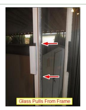
(2) Inoperative Window Locks. The window lock(s) for the windows in some of the rooms did not function. It was noted that the window did not align within the frame. For safety purposes it is recommended that this window be adjusted, repaired or supplied with some sort of locking device.
