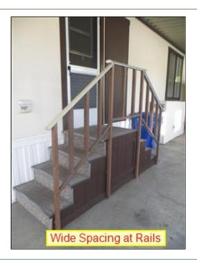
(2) Wide Hand Rail Width. The hand grip surface of the handrails at the rear of the house are currently greater than 2 inches. Handrails should have a hand grip surface of no less than 1.25 inches nor more than 2 inches in cross sectional dimension. Recommend correction of handrail width.
