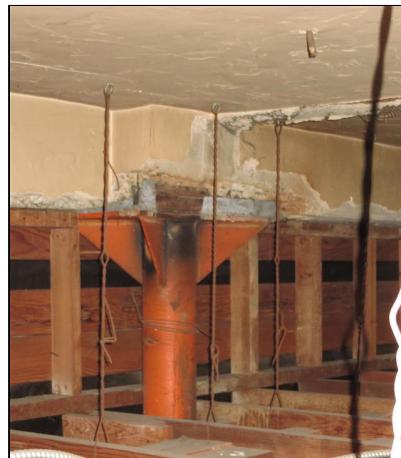
Exterior Wall Construction (Between Floors)
